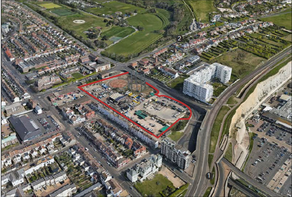
Figure 1 – An aerial photograph showing the appeal site and its context. 14
